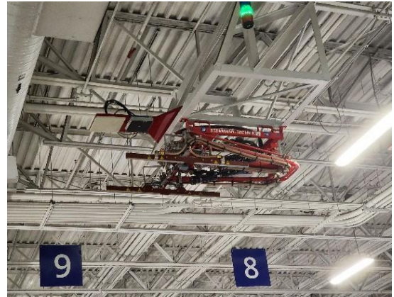
This is a picture of one of the charging devices (pantographs) which drops from the ceiling to the top of a bus. It is one of the many unique features of the state of the art garage.
